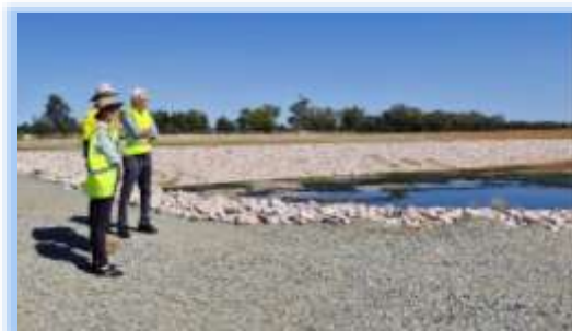
Inspecting the Treatment Ponds.
