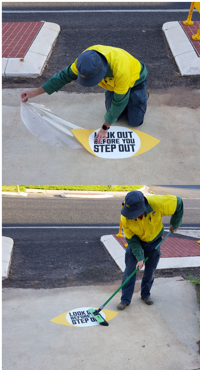
Photo caption: Installation at a pedestrian facility
