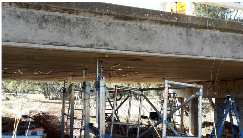
Test set up of deflection and strain measurement of Barellan Bridge for Road Train at HML
