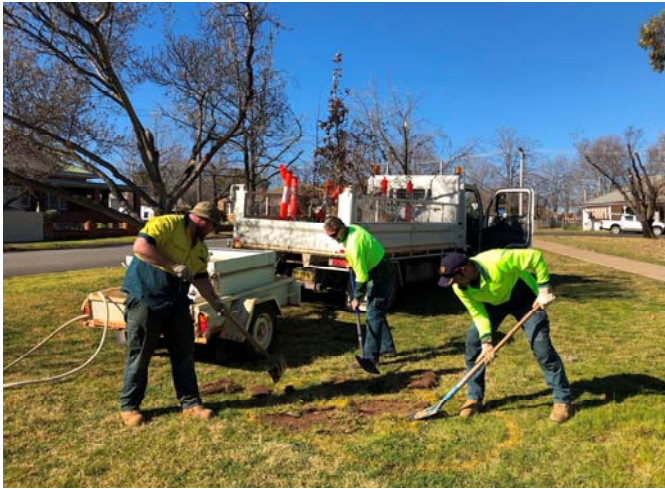
Staff preparing to plant trees at Jonsen Street Park.
