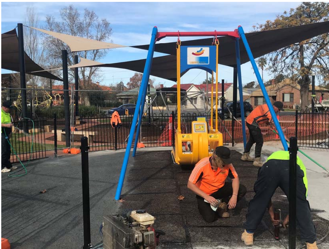
Liberty Swing construction at Marie Bashir Park.
