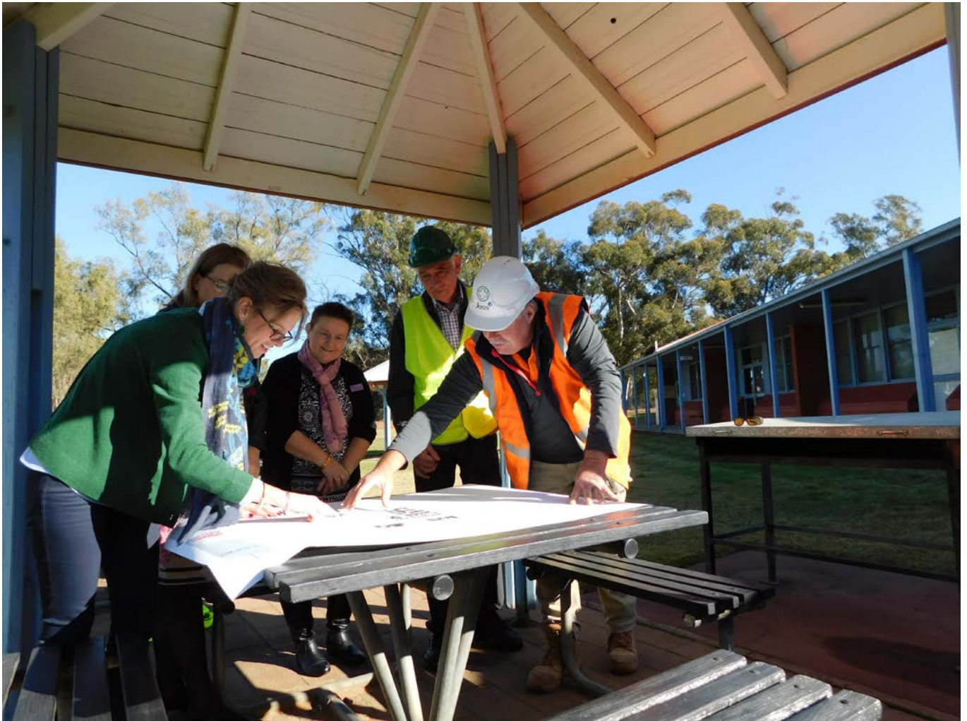
Local Member for Cootamundra Steph Cooke MP, Sara Morley, Relieving Deputy Regional General Manager TAFE NSW; Josie Marks, TAFE Services Co-ordinator for Narrandera Campus; Mayor of Narrandera Shire Neville Kschenka; and Maurice Wood, site manager for Joss Constructions inspecting the new campus layout.
